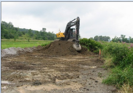
Excavating abandoned railroad bed (in black), restoring floodplain
