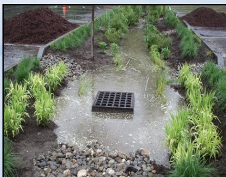
Green stormwater infrastructure receives and filters stormwater from parking lots
