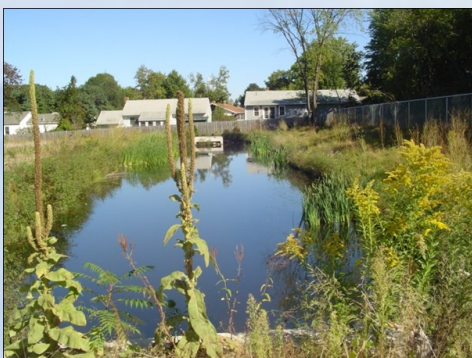
Expanded stormwater treatment pond
