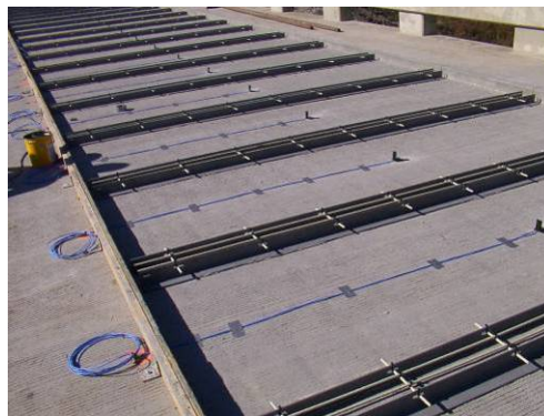
Electrode Arrangement (Tuan 2004a)
