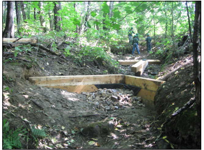
Check dams along a gully in Williston Hills
