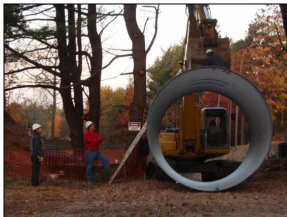
Construction at Gully C, October 2008
