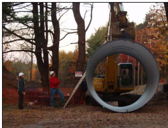
Construction at Gully C, October 2008
