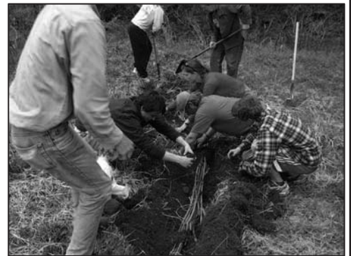
Installing a willow fascine in Worcester along the North Branch with community volunteers
