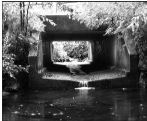
Potential culvert retrofit project in Underhill, Browns River watershed
