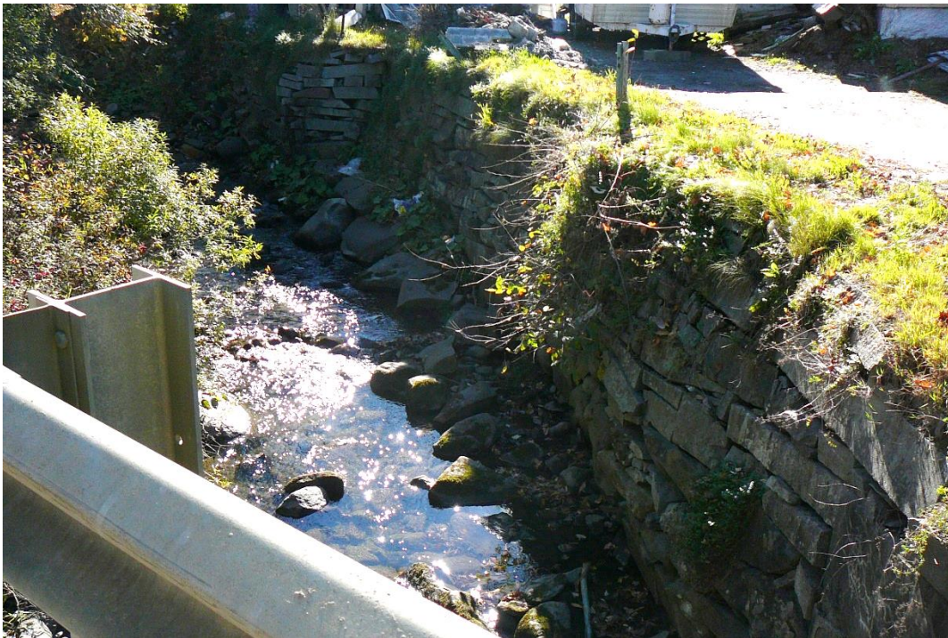
Figure 30. View of quarried stone slab retaining wall along the south bank of the Jail Branch, downstream (west) of the dam, looking southeast.
