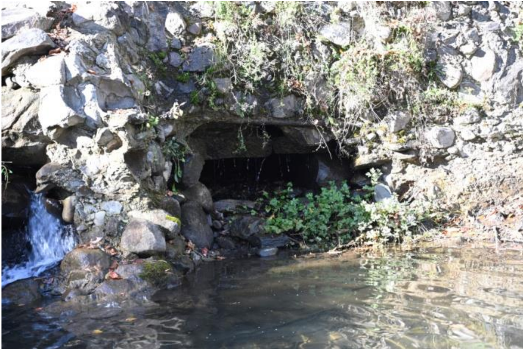
Figure 28. View of the tailrace outlet built into the turbine pit structure, looking west.
