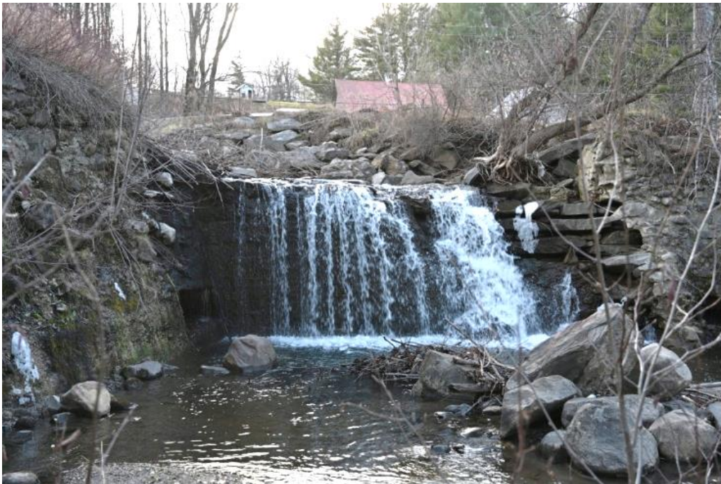
Figure 24. View along the downstream face of the spillway section of the dam (left) at the mill structure (where the water is now flowing), looking west southwest. Note location of the low outlet at the base of the spillway section of the dam, and granite grout fill and parking area visible in the background that covers part of the mill structure as well as the left wing and abutment area of the old dam.
