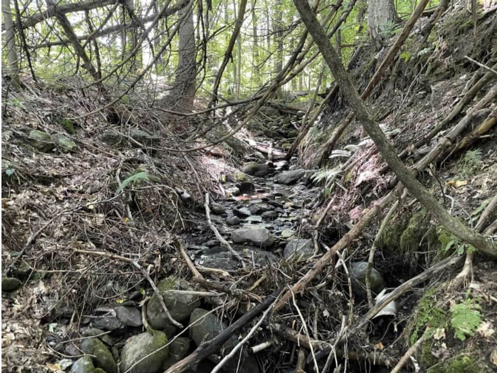
Figure 3: Project 3 – remove berm and restore gully
