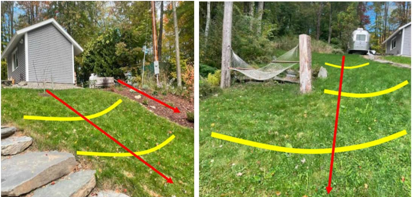
Figure 63: Project 56 – Filter berms at 452 Southwest Shore Road (photos from WNRCD)
