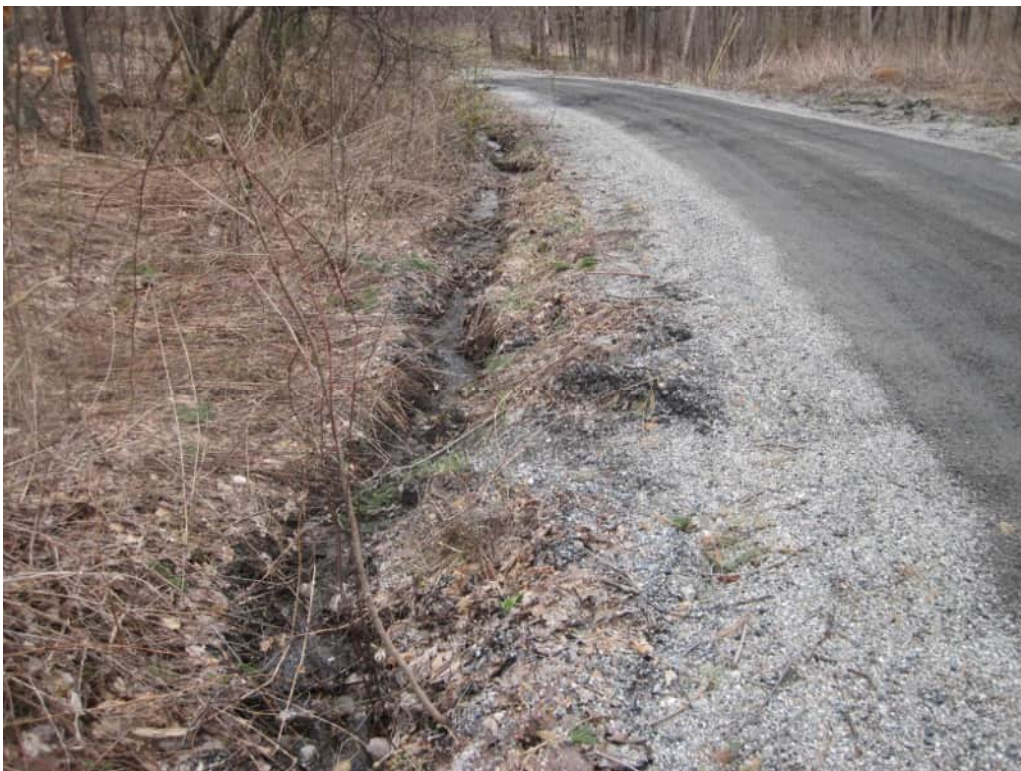
Figure 24: Project 22 – Dynamite Hill Road improvements
