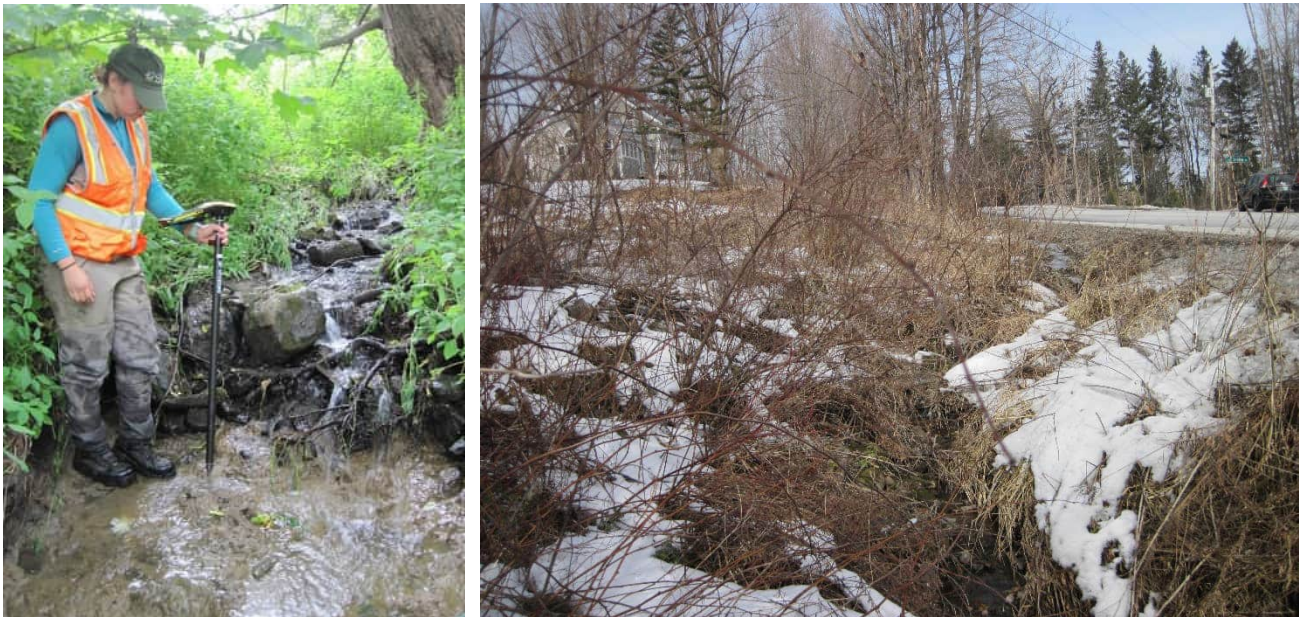
Figure 72: Project 67 – Upper Shadow Lane Tributary restoration
