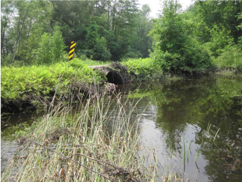
Figure 15: Project 13 – culvert replacement at Beebe Lane
