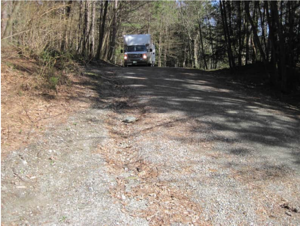
Figure 21: Project 20 – new swale along Firefly Lane
