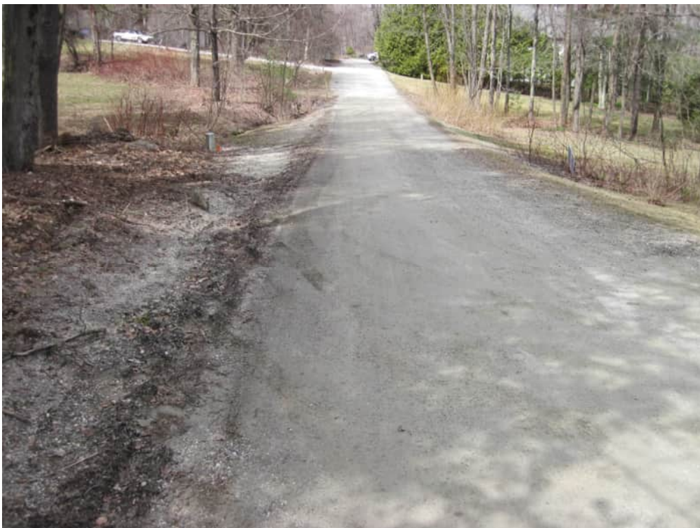
Figure 30: Project 25 – Pine Shore Drive improvements
