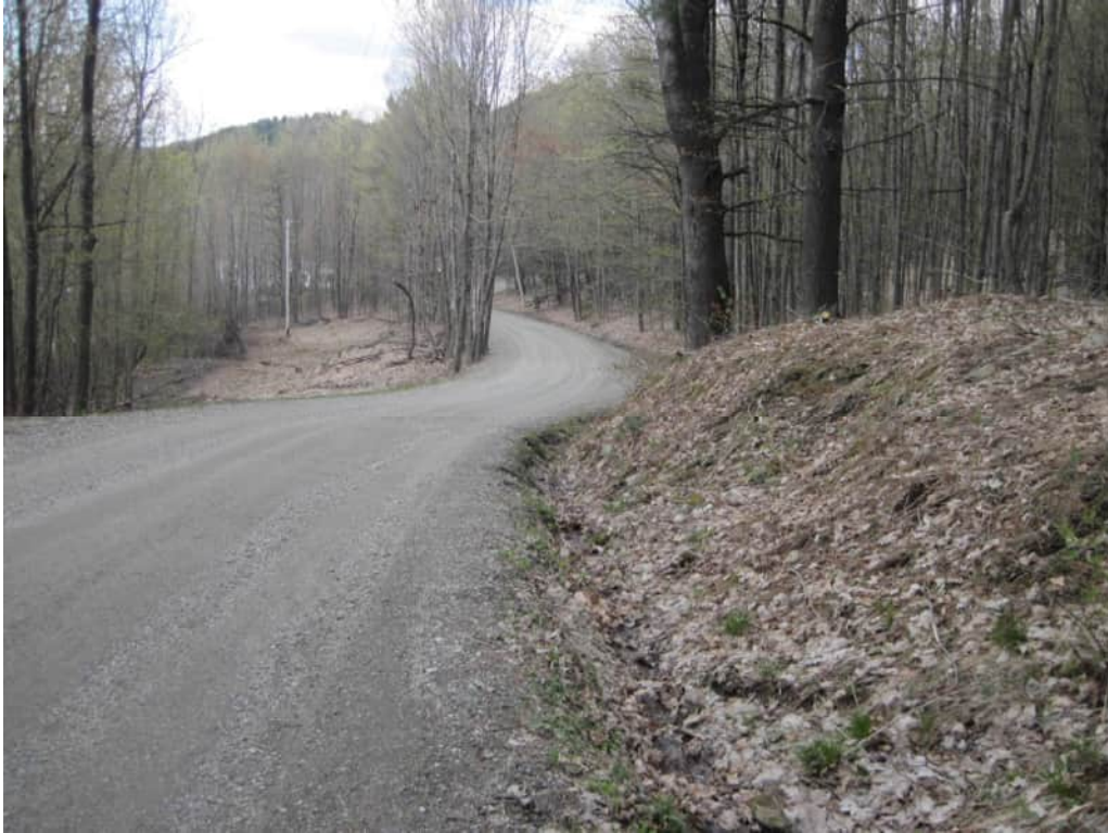
Figure 53: Project 46 – Butternut Lane improvements
