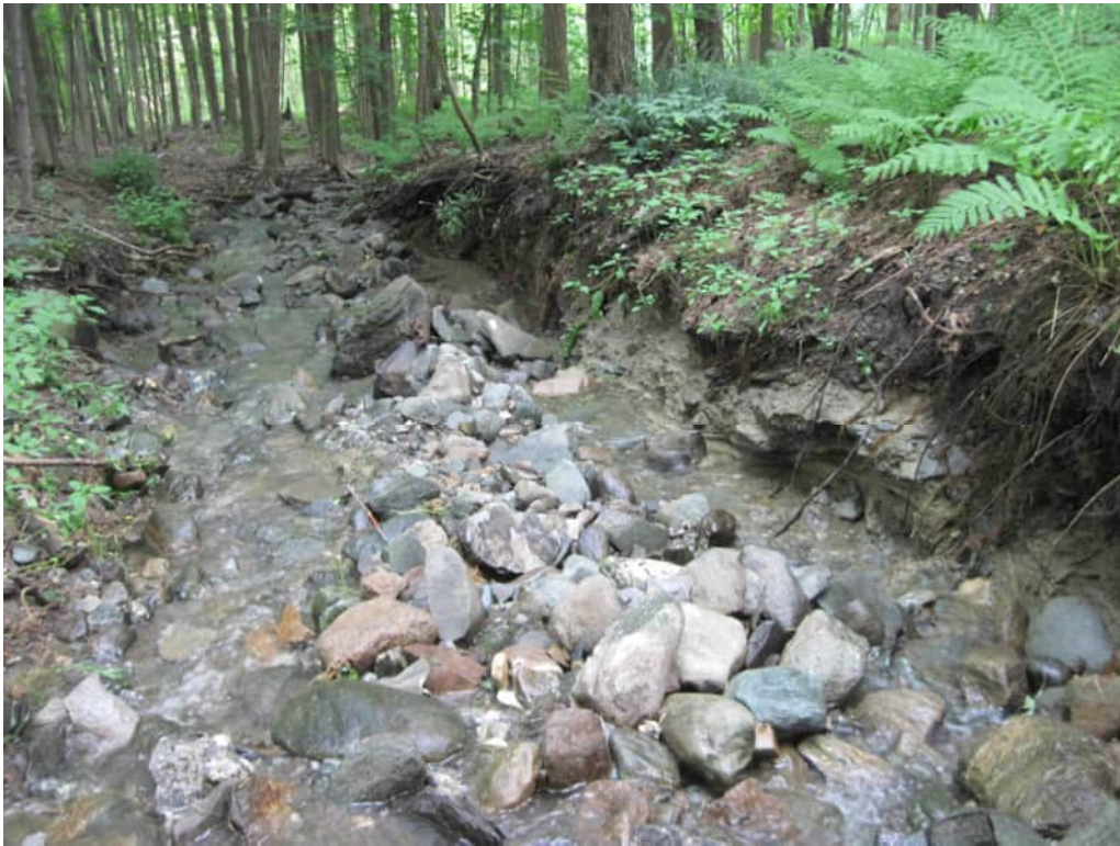
Figure 17: Project 15 – stabilize gully in Shadow Lane tributary
