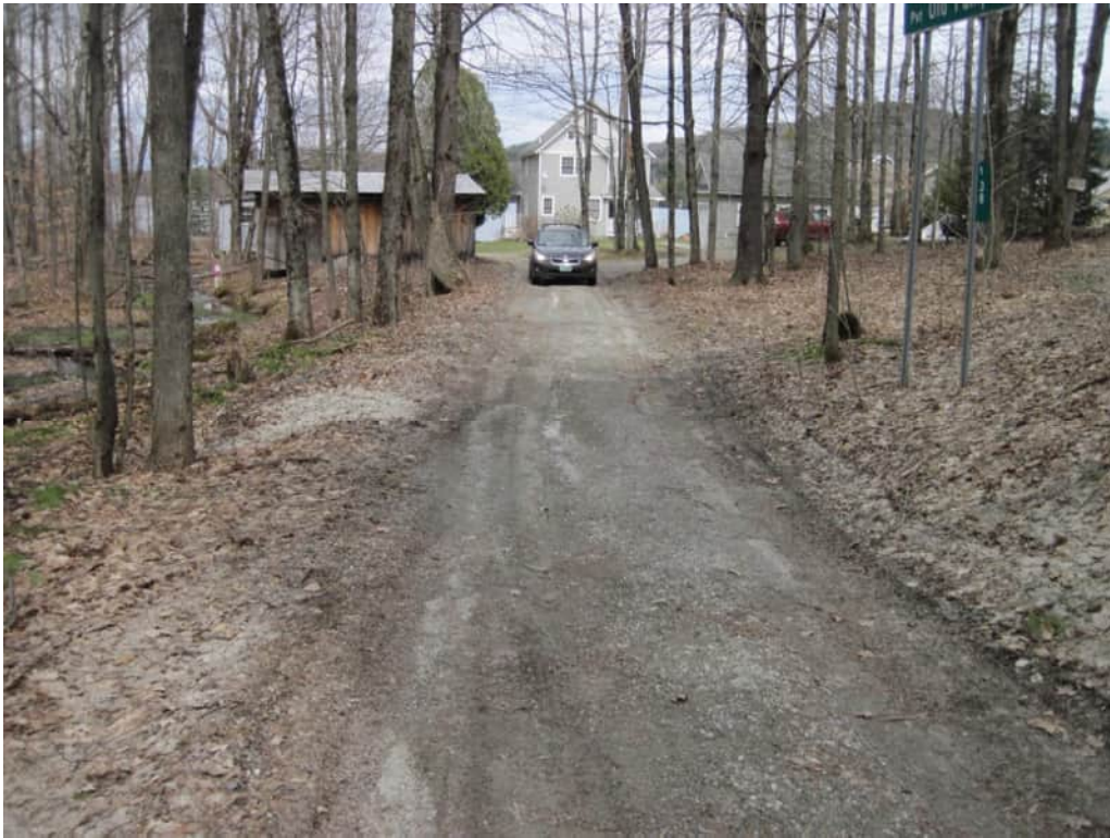
Figure 35: Project 29 – Old Pump Road improvements
