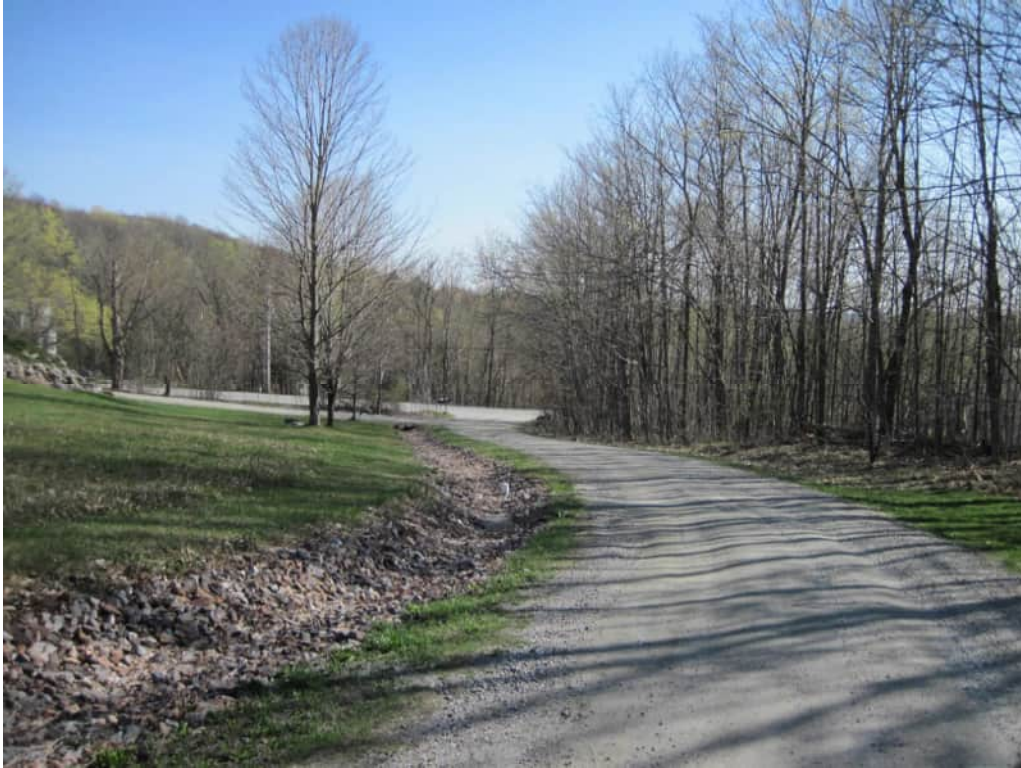
Figure 47: Project 42 – Longmeadow Road improvements
