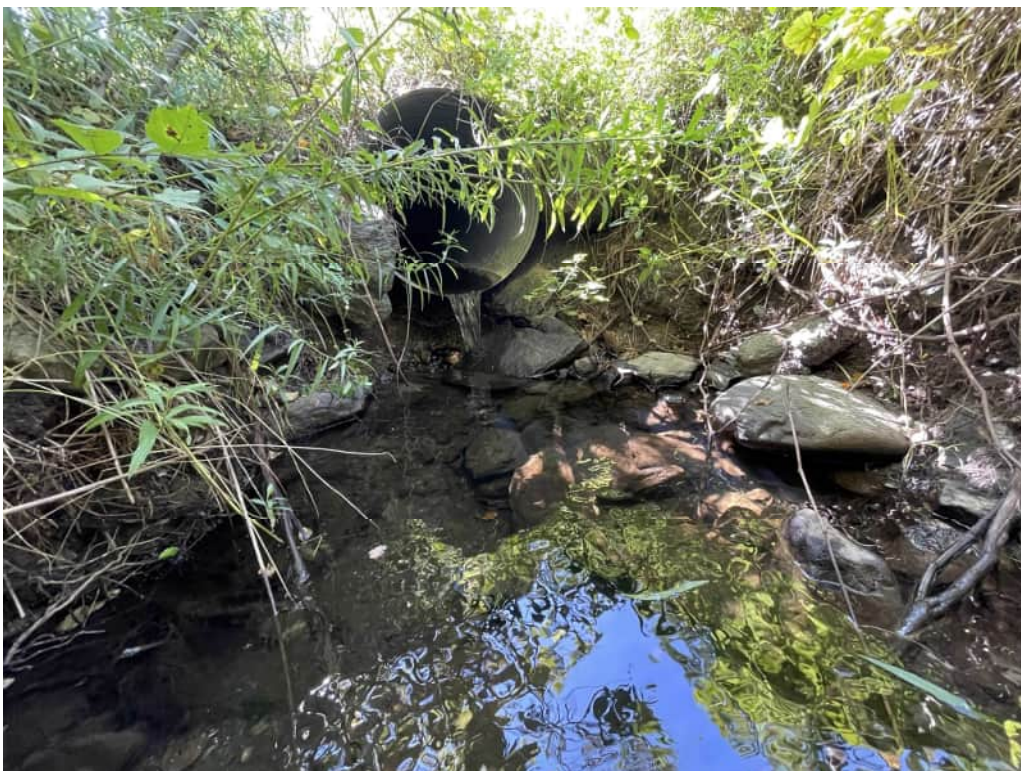
Figure 2: Project 2 – culvert replacement at Richmond Road
