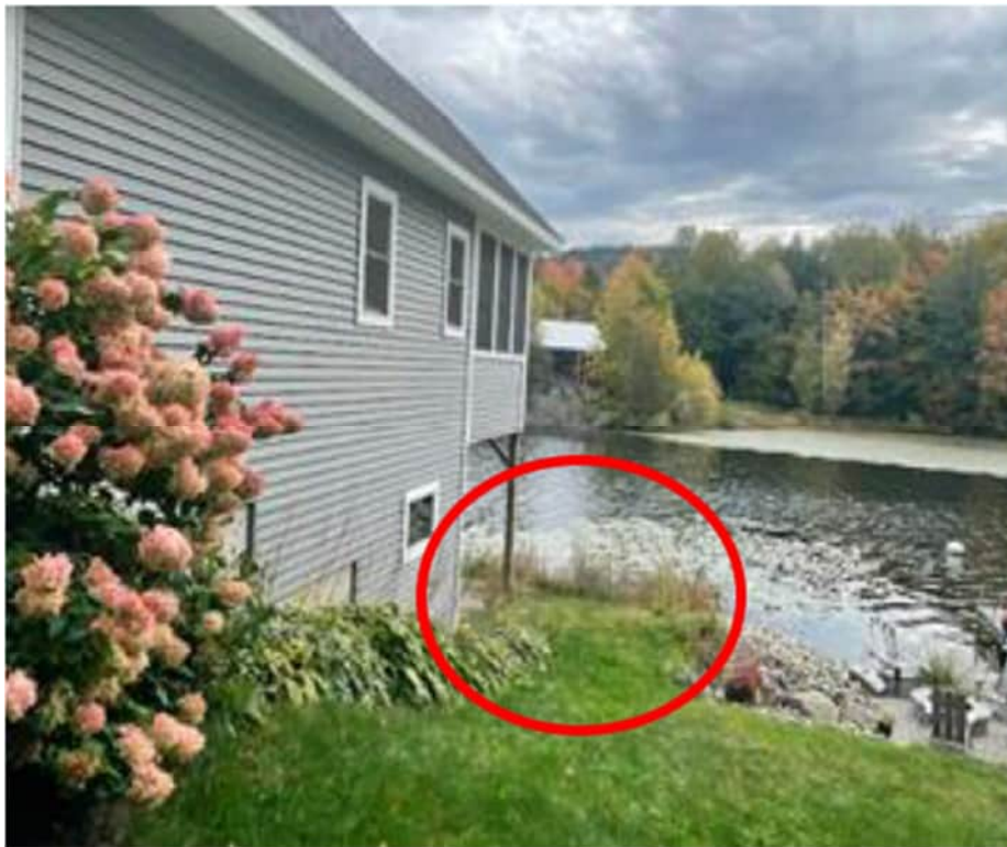
Figure 58: Project 51 –Southwest Shore Road rain garden (photo from WNRCD)
