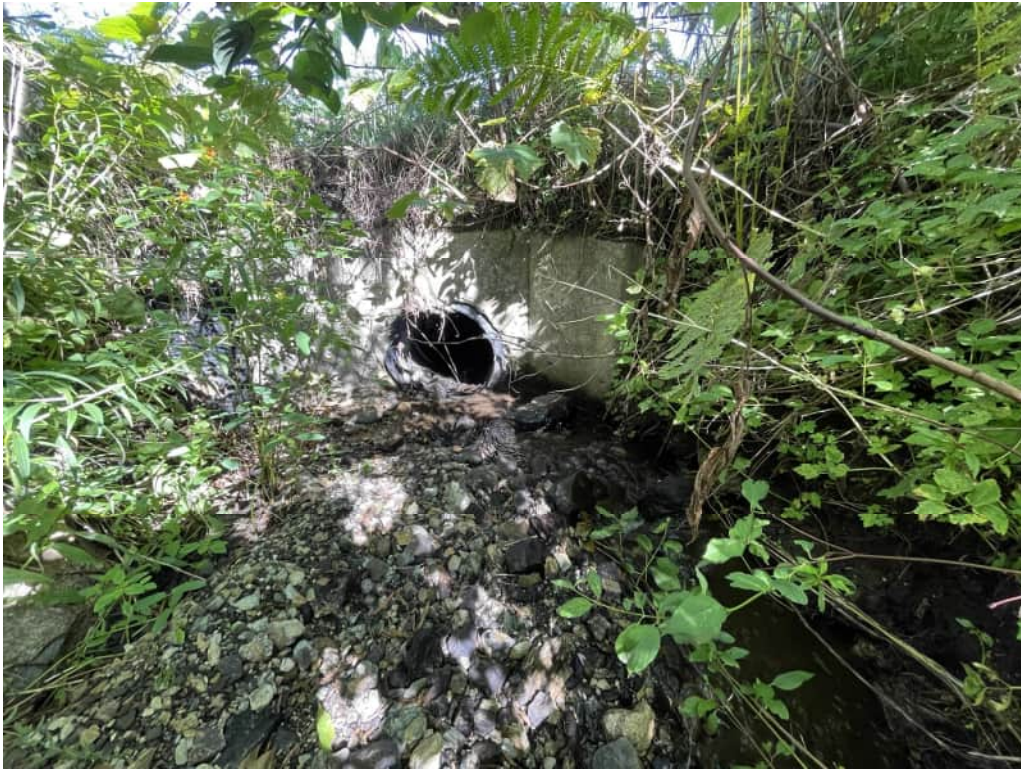
Figure 1: Project 1 – culvert replacement at Sunset Lake Cooperative
