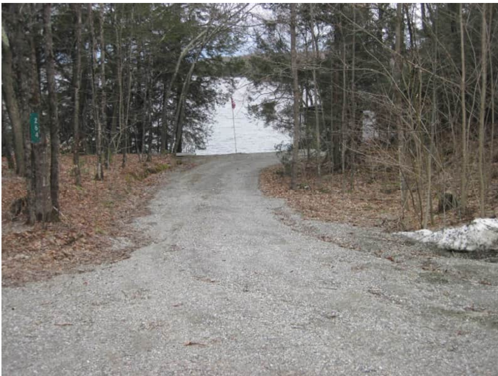
Figure 36: Project 30 – Upper Access Road improvements
