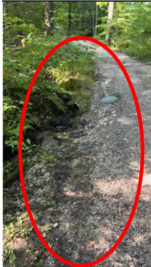
Figure 67: Project 60 – Driveway improvements at 1140 Beebe Lane (photo from WNRCD)
