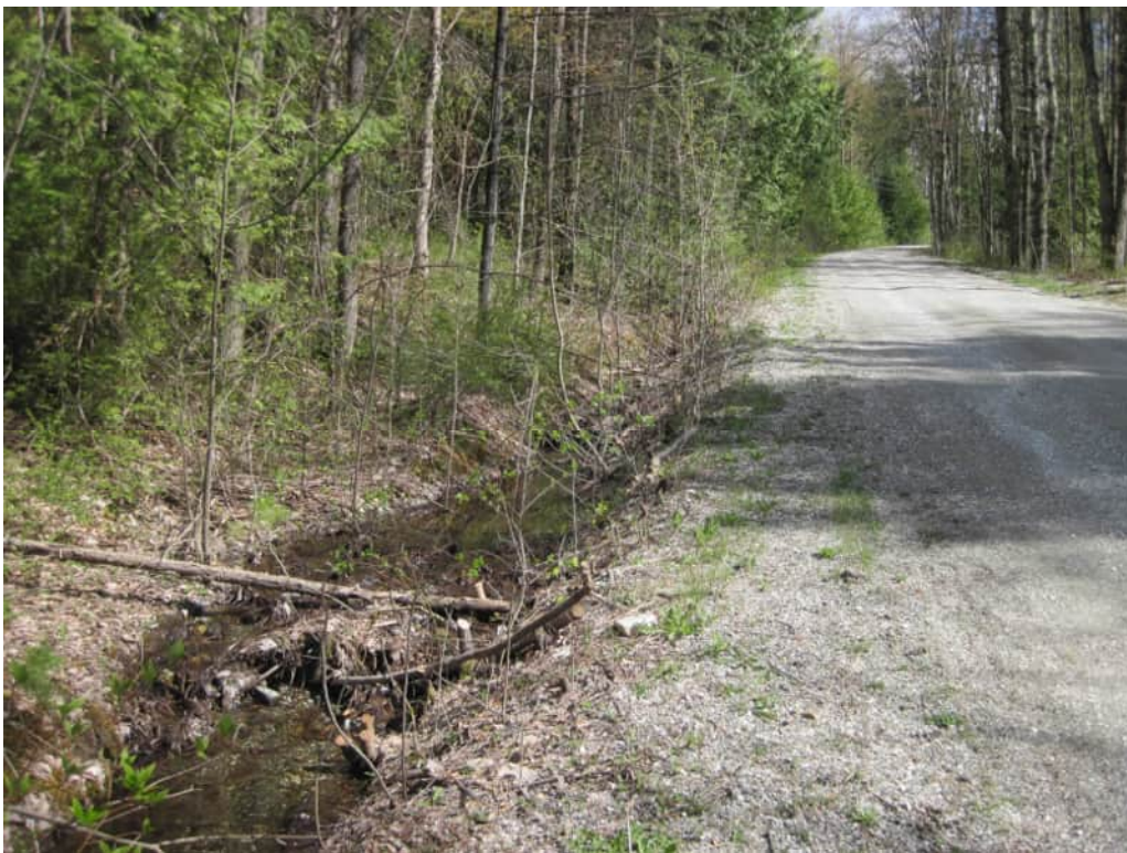
Figure 48: Project 43 – Red Pine Lane improvements
