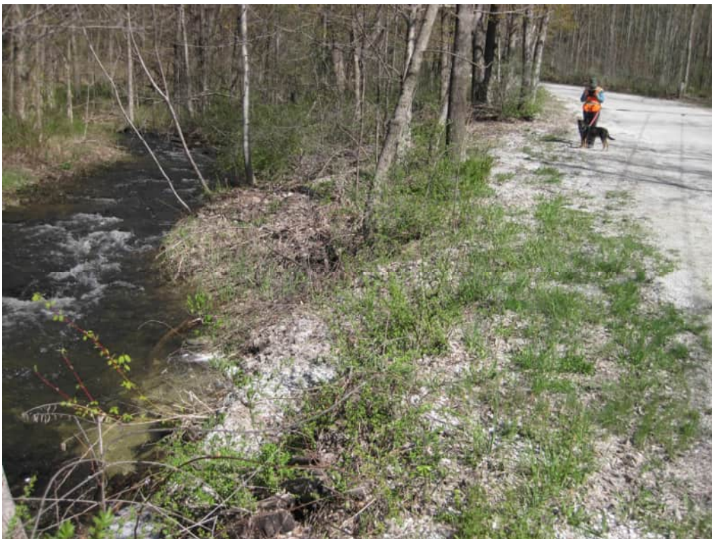
Figure 50: Project 44 – Partridge Hill improvements
