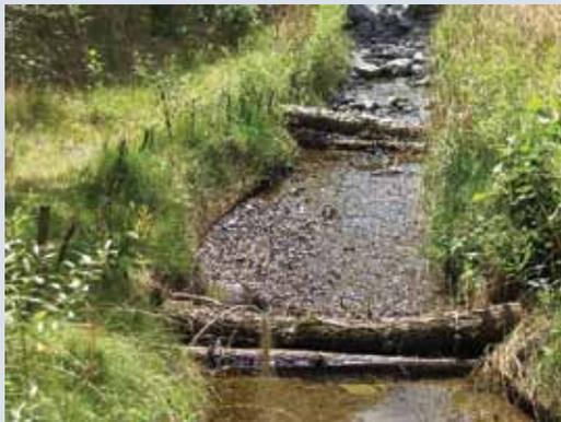
*Cascade (above) with excavated floodplain at lower end of project site to arrest the headcut and restore floodplain function. At right, re-established riparian vegetation.*
