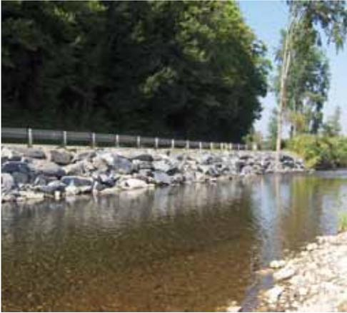
*A road is located in close proximity to the river. Along with negative impacts of failed riprap along the banks, it also becomes expensive to continue to maintain riprap to protect infrastructure that is placed in the river's meander path.*
