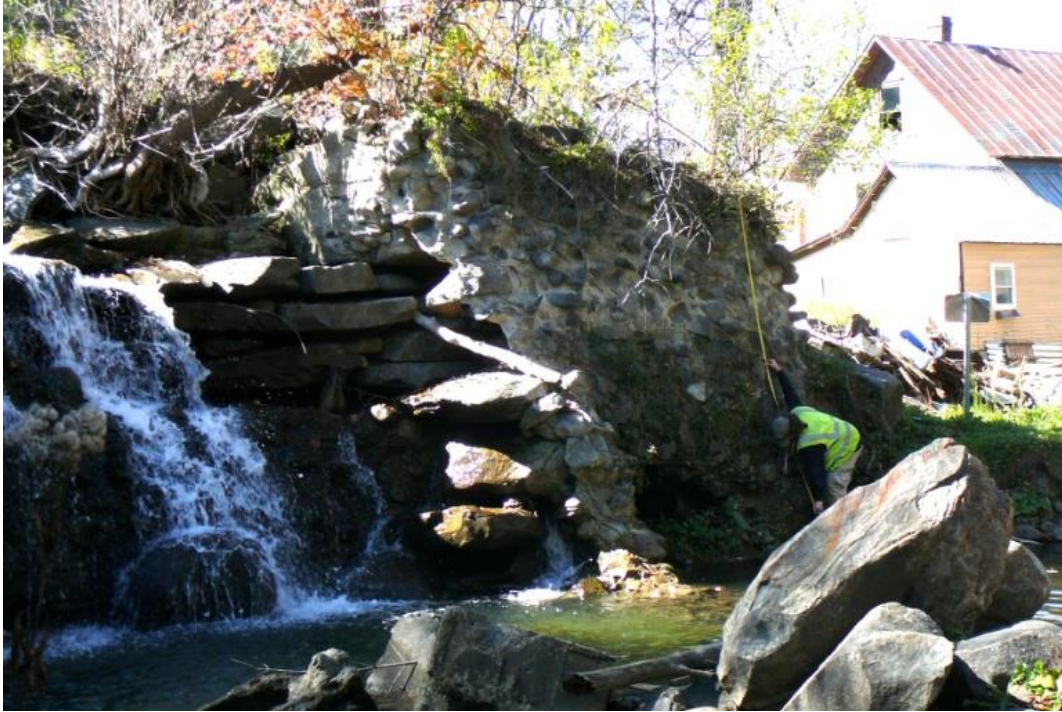
Figure 29. View of the turbine pit structure associated with the mill building, showing the rough stone and concrete ‘shell’ around and above the older structure, looking northwest.
