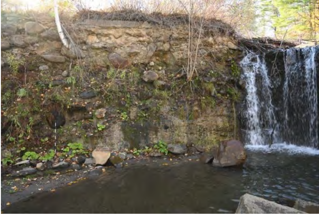
Figure 18. View of the left part of the Hands Mill Dam spillway, looking southwest. Note: top section of the spillway appears to be either a different concrete or a different lift, minimal amount of original surface remaining on the downstream face of the structure, and the exposed interior of the rubble / cyclopean concrete.
