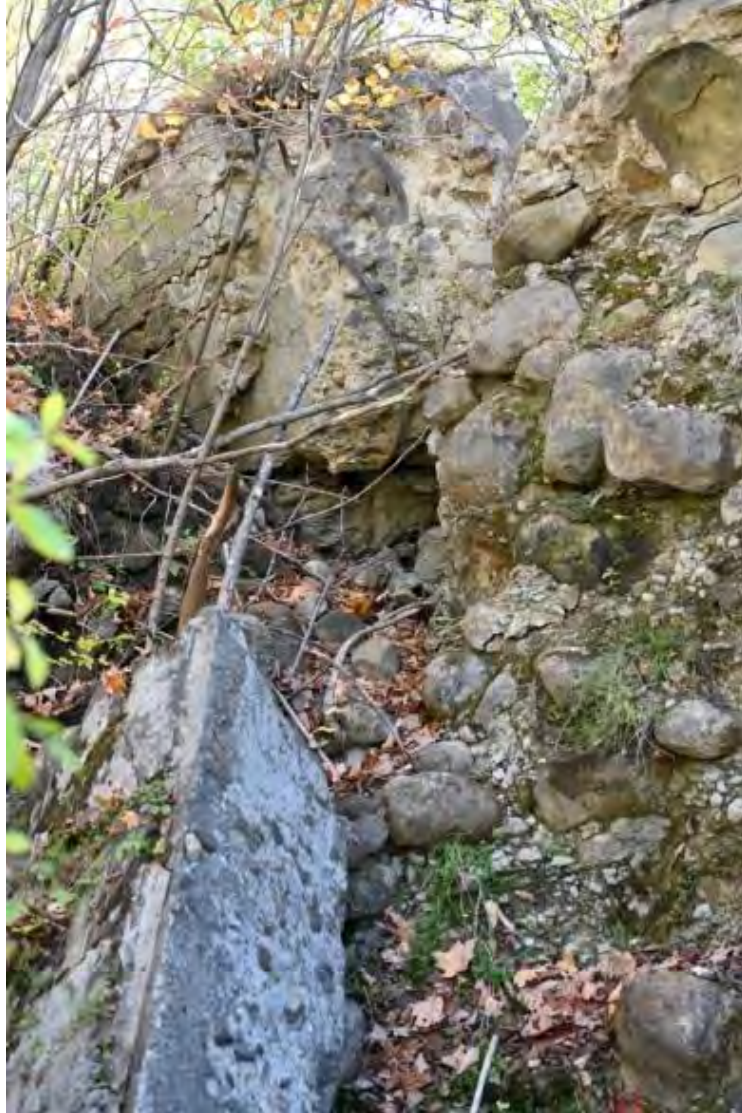
Figure 22. View of the compromised joint section between the spillway (closer) and the right wing sections of the dam, looking east southeast. The right wing structure is formed of rubble concrete and contains some metal reinforcement, possibly plain round bar and flat scrap metal pieces; this part of the structure also appears to have had another layer of concrete (a facing or a veneer) on its downstream side (two board formed surfaces appear to be visible).
