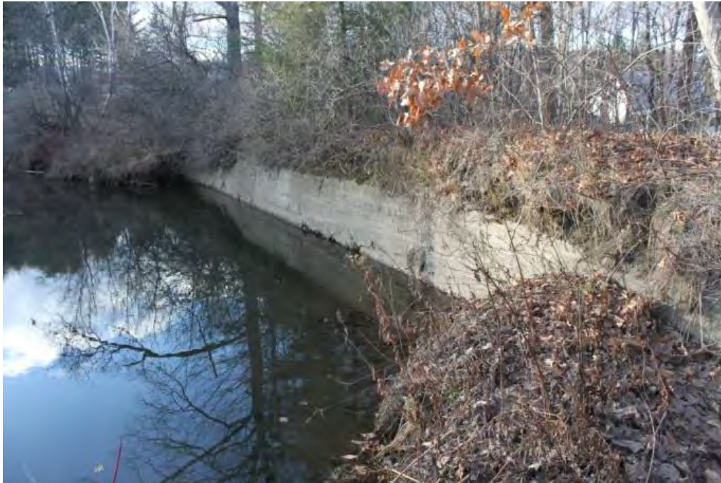
Figure 23. View looking west along the upstream face of the right wing wall / cutoff wall looking towards the spillway section of the dam.
